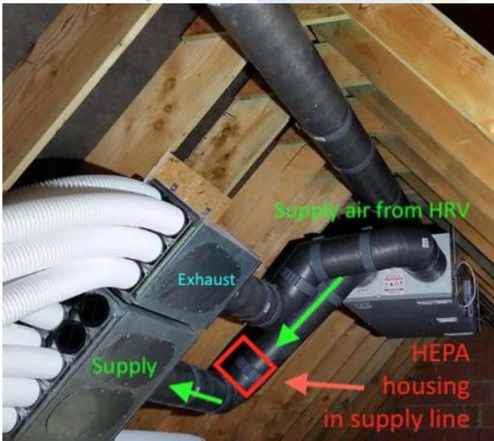
The system was balanced when commissioned and has been running beautifully. I do not show all aspects of the installation and am just focusing on the supply side and HEPA install.
